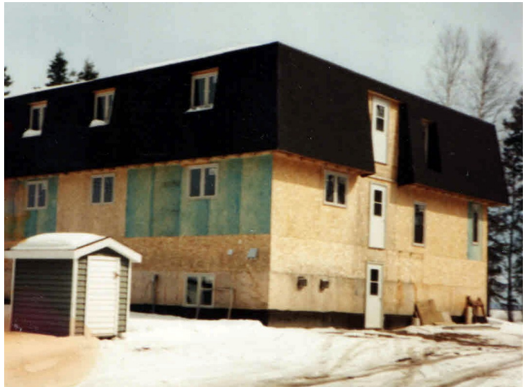
Eagles Nest under construction
